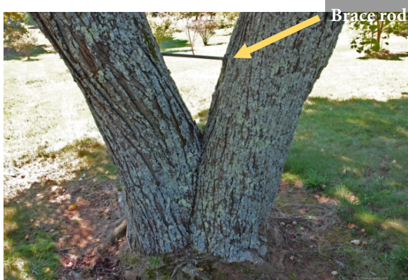
Figure 2: Brace rods are installed low on the branch and below the junction if a crack is present
