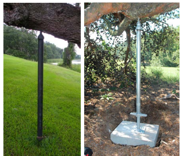
Figure 2: Finished "I" prop (left) and prop system showing anchoring and height adjustment (right)
