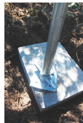
Figure 8: Lower the support nut on the jack to the lowest point and insert into the pipe
