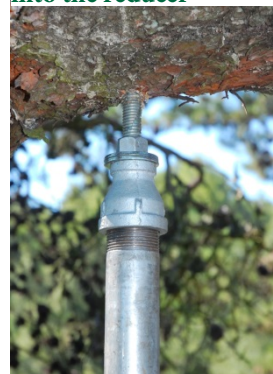
Figure 9: Screw the pipe into the reducer
