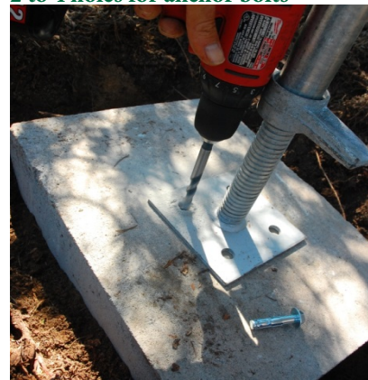
Figure 10: Use a masonry bit to drill 2 to 4 holes for anchor bolts
