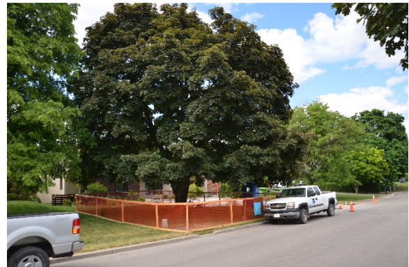
Figure 2: Construction barriers installed to reduce damage to roots and soil
