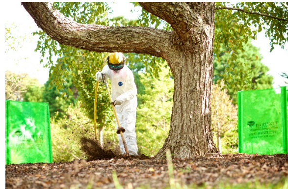
Figure 1: An AirSpade® is loosening soil and incorporating organic matter for a shade garden planting
